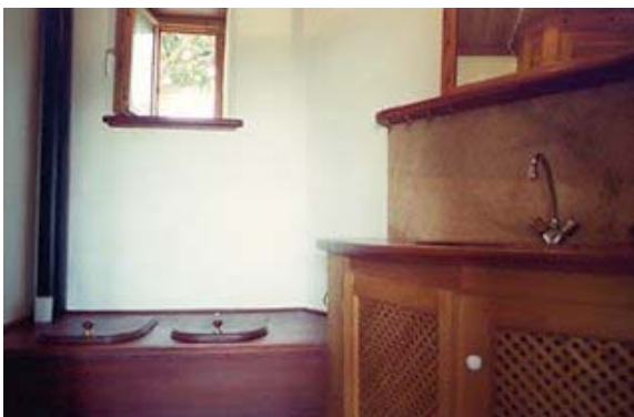
Figure 10 : Dry toilet integrated in the bathroom Source: www.rinconesdelatlantico.com
