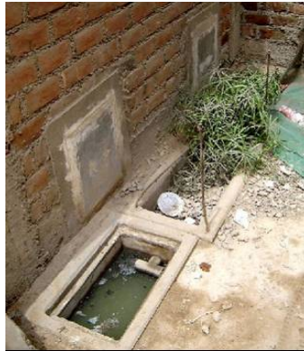
Figure 2: Until 2007 UDDT in Lima always mixed greywater with urine, the infiltration often didn't work properly Source: P.Oswald
