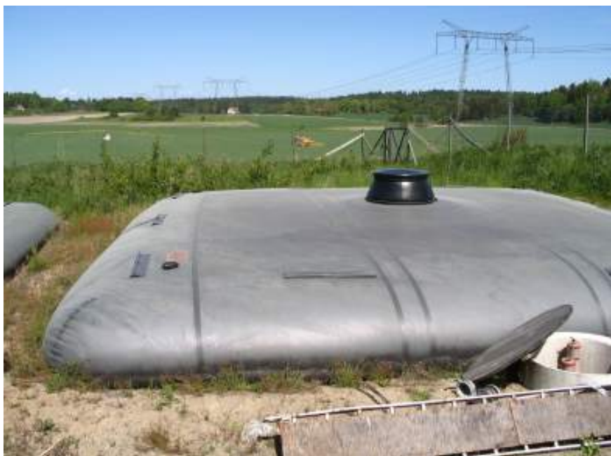
Figure 12: Urine storage at Bornsjön, Sweden (Source: P. Jensen)
